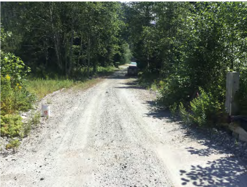
Left Approach Facing Away From Bridge
