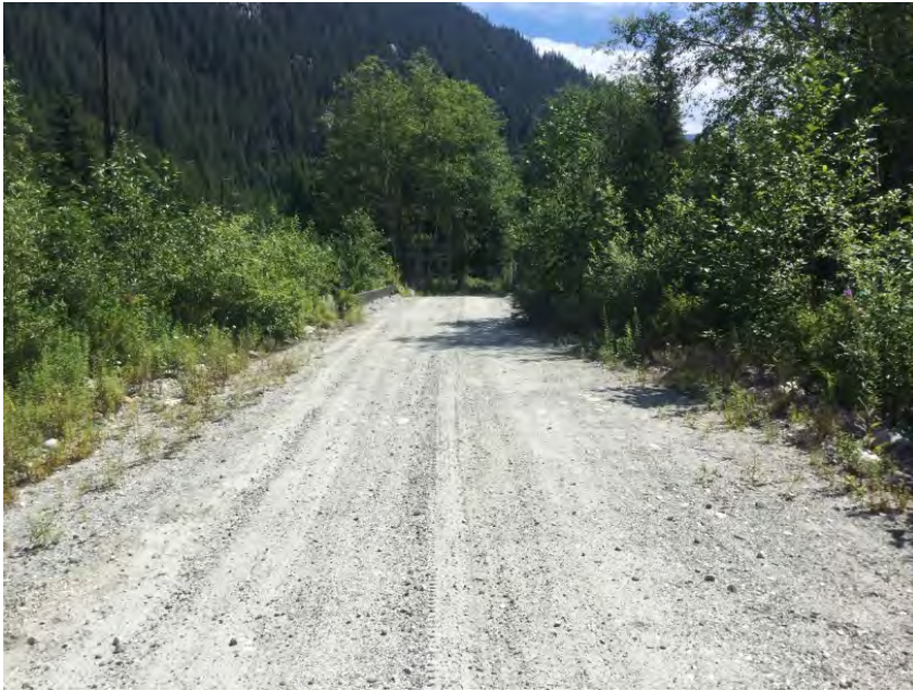
Right Approach Facing Bridge
