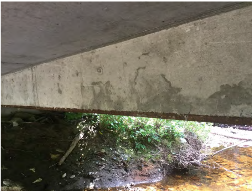
Girders Monolithic with Deck
