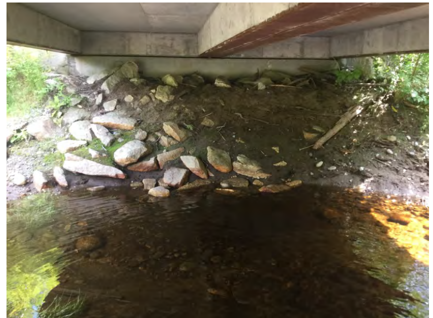
Left Bank Abutment
