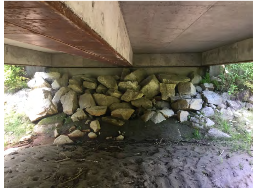
Left Bank Abutment
